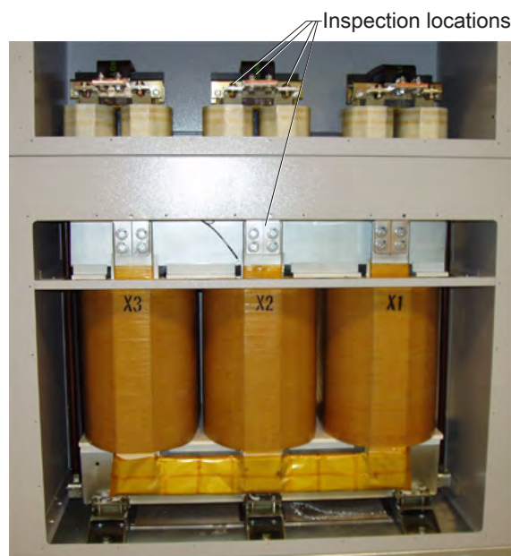
Figure 4-5. Inductor and transformer connections
