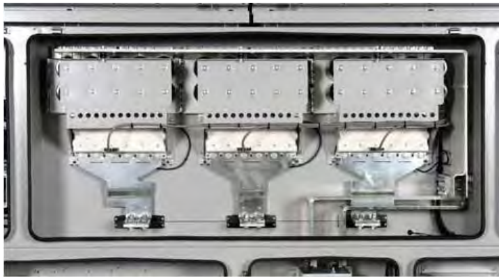
Figure 2-2. Power module assembly
