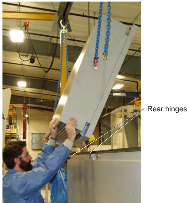
Figure 4-2. Placing the air intake hood on the inverter
